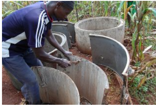
Removing the concrete rings from the molds.
