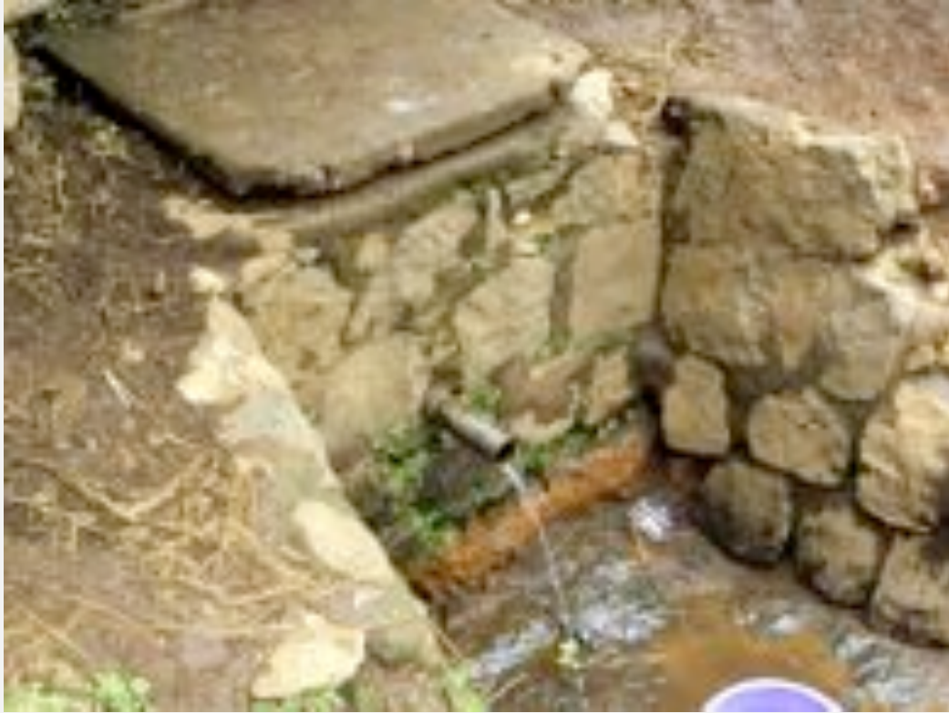
The old Takui water tap (above) was dirty and poorly managed. Without a catchment container, the water flowed constantly during the rainy season and was often dry during the dry season.
