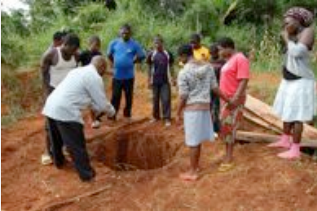
A rural engineer and Jakiri residents examine the freshly dug (by hand!) hole for the well.
