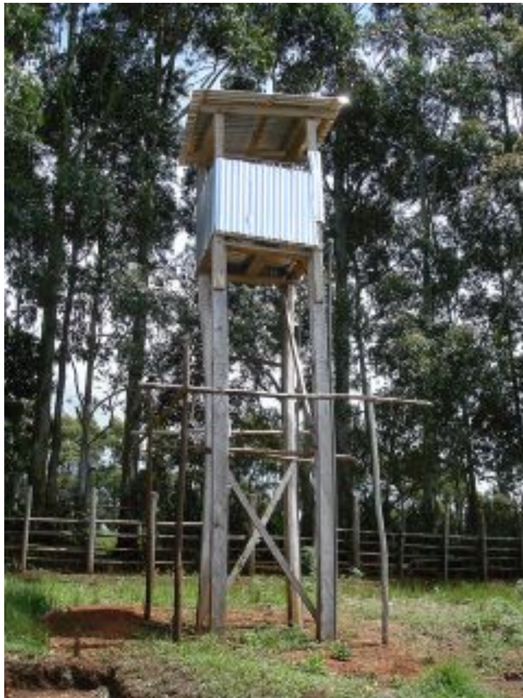
The water storage tank at the top of the land is elevated on a tower to increase water pressure for the roadside and irrigation taps.
